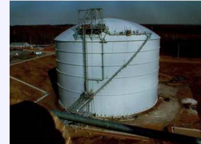
**Storage:** LNG is stored in double-walled, insulated tanks at atmospheric pressure. These tanks are designed to prevent any leaks. There is also a dike around the wall that is capable of containing the entire volume of the tank in the unlikely event of a spill.
