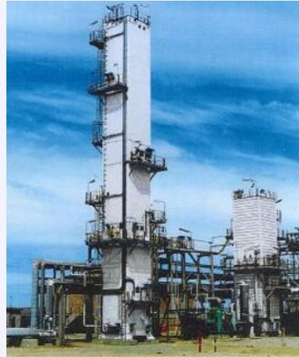
**Liquefaction:** Gas from the production field comes to the liquefaction plant. Contaminants are removed and the gas is cooled to a temperature of  $-256^{\circ}\text{F}$ . By liquefying the gas, its volume is reduced by a factor of 600.
