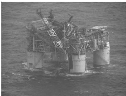
The Mars tension-leg platform after Hurricane Katrina.
